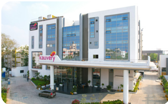
MAA KAUVERY HOSPITAL Trichy, Cantonment
